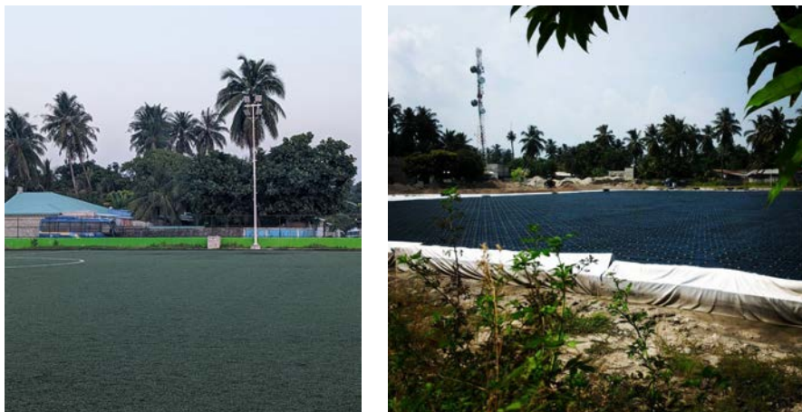
Figure 8: Current ZigZag stadium under which aqua cells are located (left), and aqua cells during construction phase (right)
