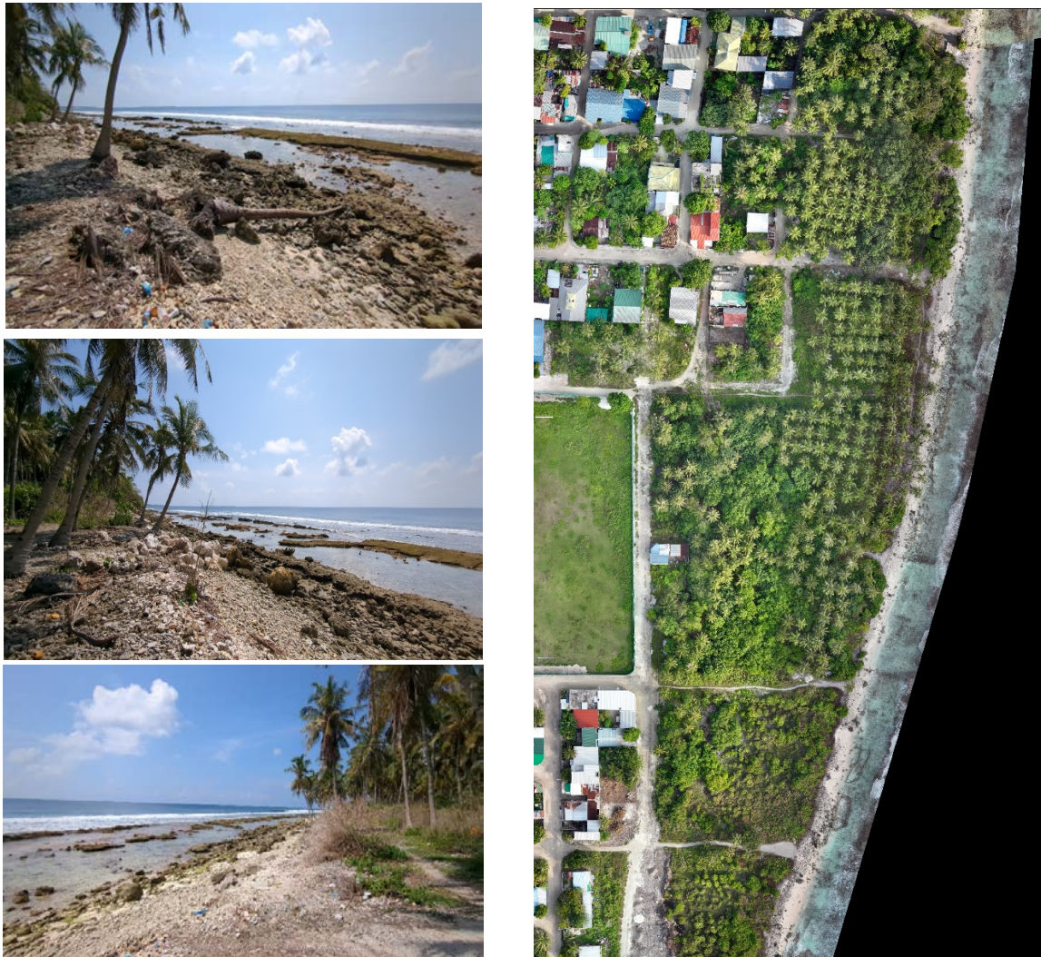
Figure 25: Current status of the eastern shoreline: south-central section
